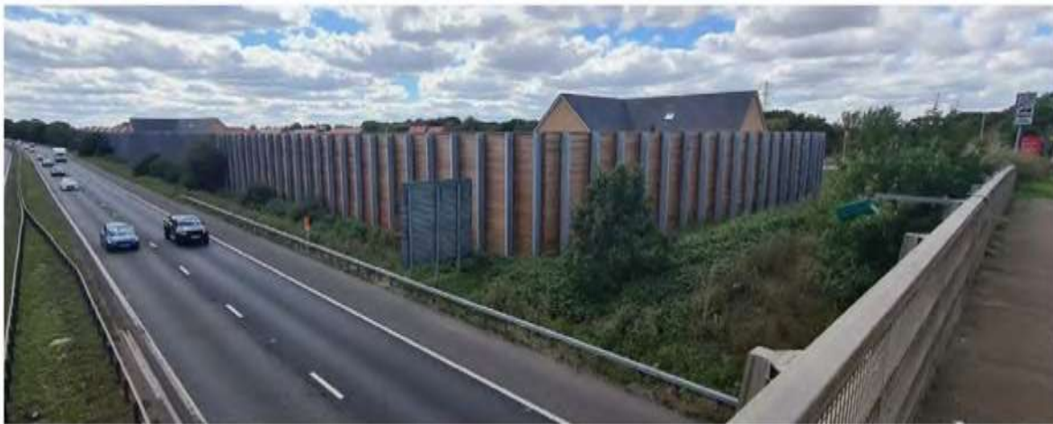
Figure 7 - The noise barrier as viewed from Fishers Green Lane Bridge with the new housing beyond plus the northbound carriageways of the A1M.
