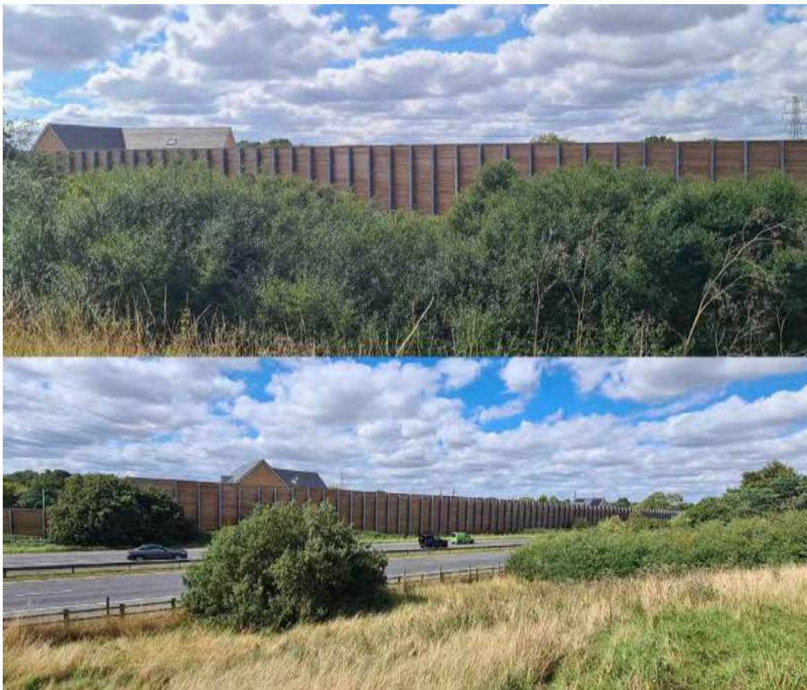
Figure 8 - Part of the noise barrier viewed from the mound on the eastern side of the A1M and south of Fishers Green Lane bridge. This mound is the primary screen of noise to the east side of the road.
