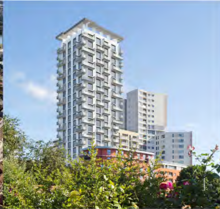
226-244 High Road (2015) Ilford Matthew Lloyd Architects
