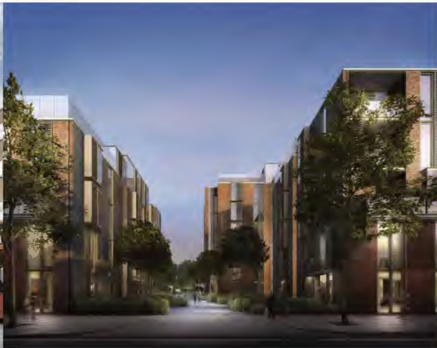
Hurlingham (2013) London Borough of Hammersmith & Fulham Hopkins Architects
