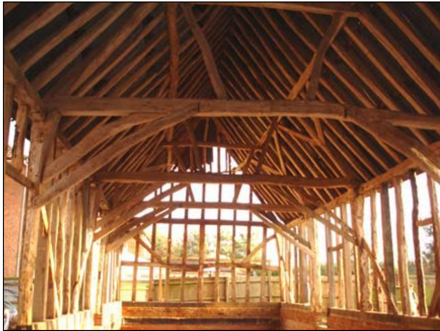
Figure 20. Oakfield Barn, timber frame undergoing repair
