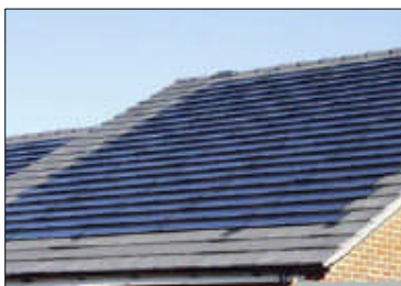
Photovoltaic panels installed on a residential property. The cells are designed to integrate with the roof tile.
