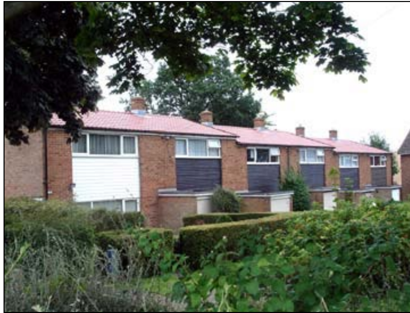
Figure 32. Red plastic 'tile-effect' replacement roofs on Burydale
