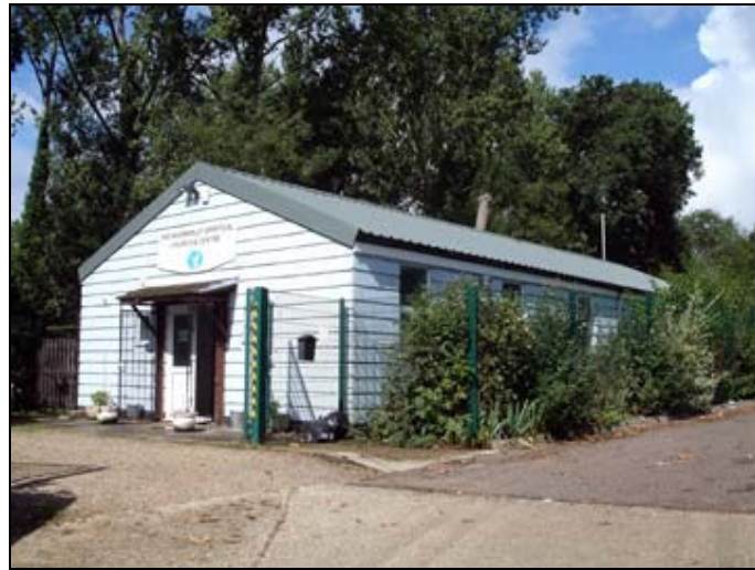
Figure 24. Whomerley Spiritualist Centre; an example of ‘Butler Block’ construction
