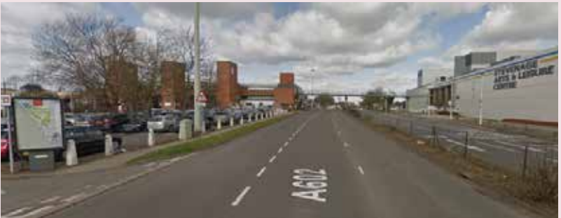
Figure 7: View of Lytton Way from south
