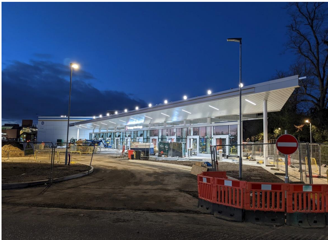
Stevenage Bus Interchange (Under Construction)
