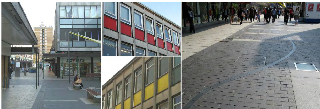
Figure 10 Timber clad canopies with steel supports (l), coloured pre cast panels (c) and block paving (r)
