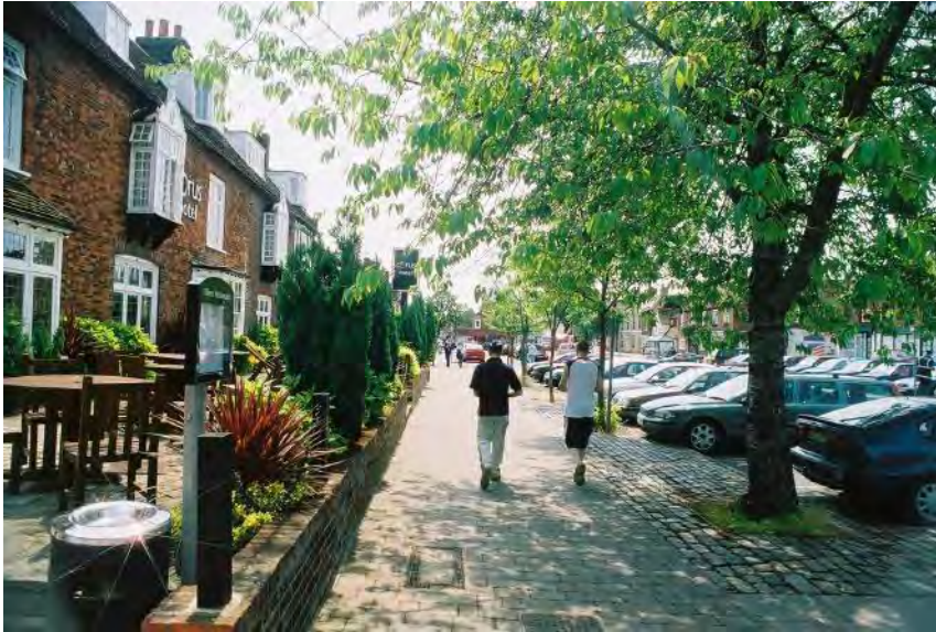
Figure 27 The Old Town High Street is the oldest conservation area designation in Stevenage
