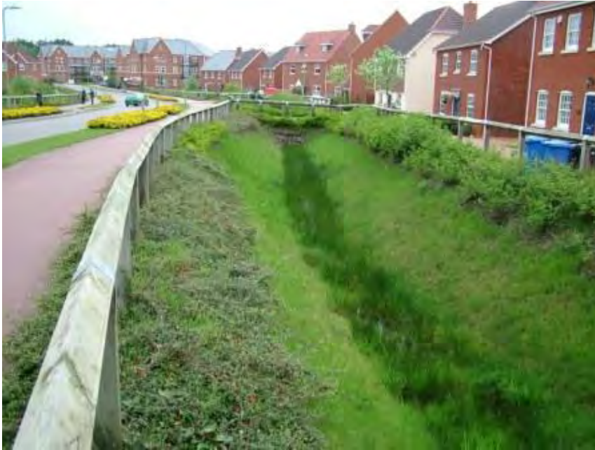
Figure 23 Drainage channels built into new developments are an example of a SUDs scheme. A flood adaption measure.
