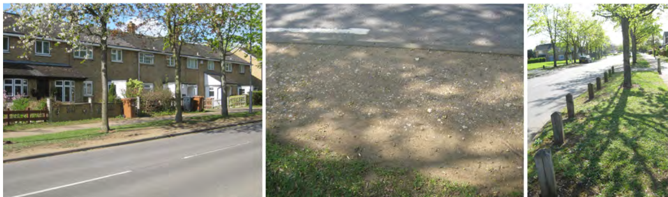
Figure 8 Damage to the grass verge caused by parking
