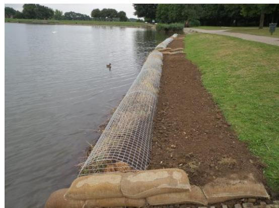
During installation, gaps were intentionally left between the coir rolls to enable WGCAC to install fishing platforms, or swims. The platforms serve to improve fish health by discouraging 'dragging' of fish onto the bank.
