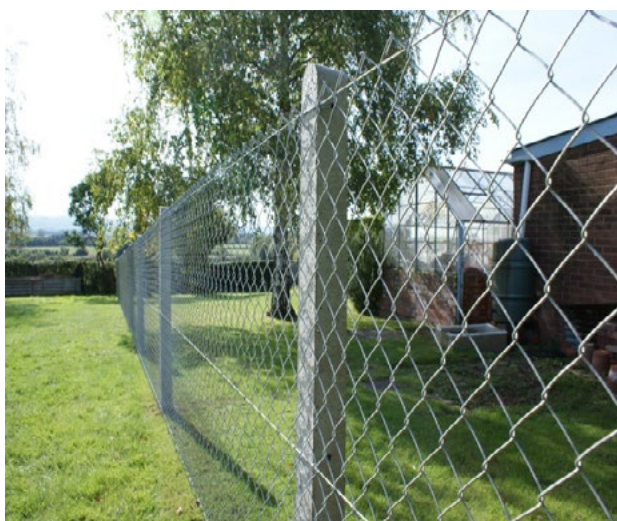
Picture 1 - Chain Link Fencing
