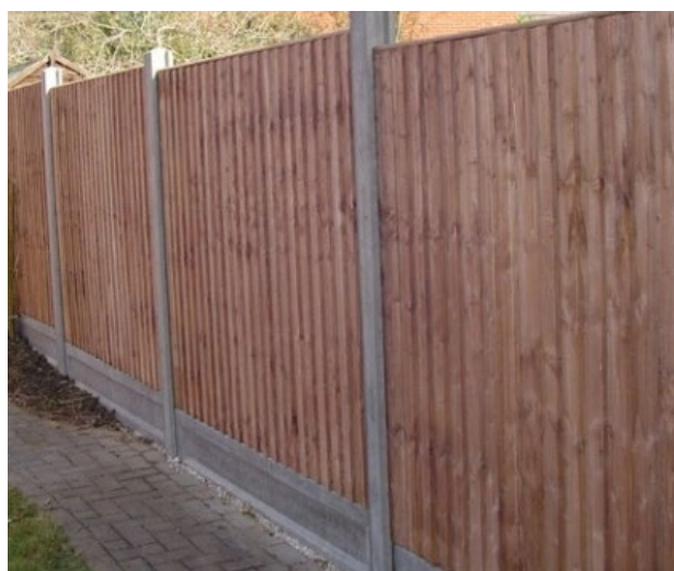
Picture 2 - 1.8m Panel Fencing with Concrete Post
