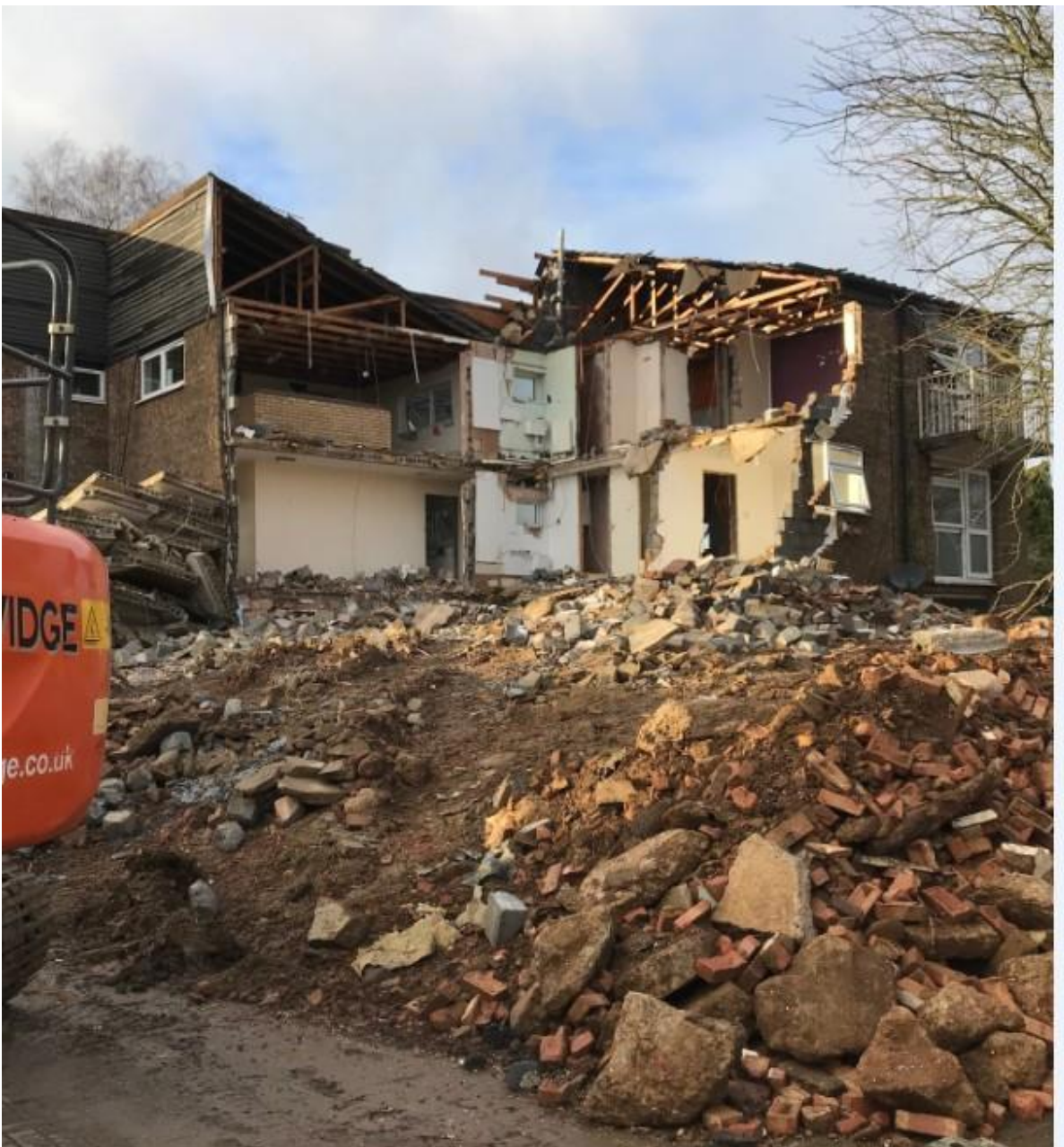
Demolition and site clearance for new homes at Kenilworth (Stirling Close)
